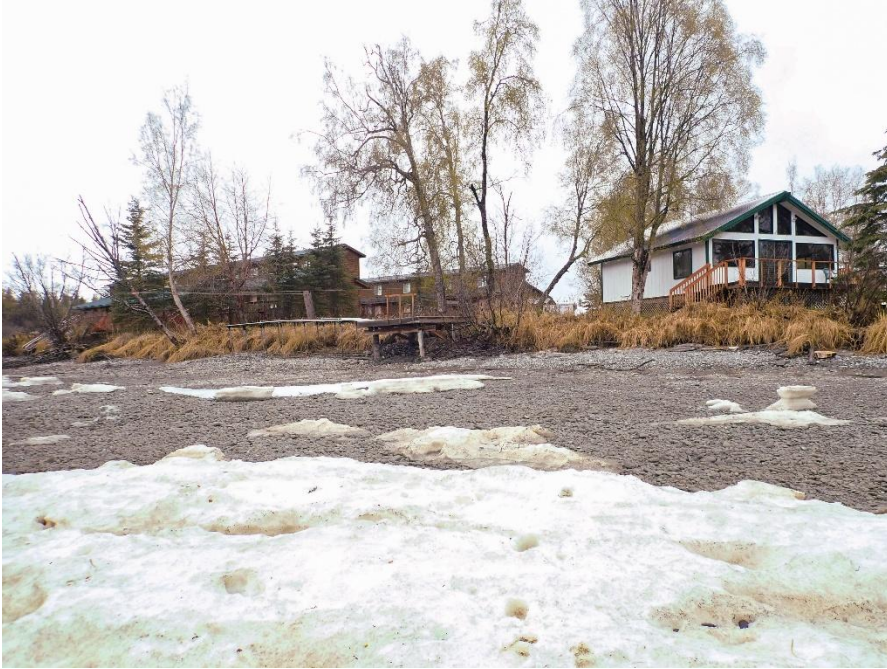
Figure 16. Pre-construction looking at the bank at site 202341, May 2022.
