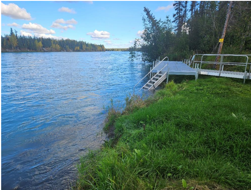
Figure 9. Post-construction looking at the bank of site 202519, September 2025.
