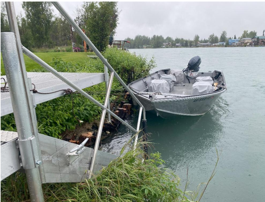
Figure 13. Post-construction looking downstream at site 202526, July 2025.
