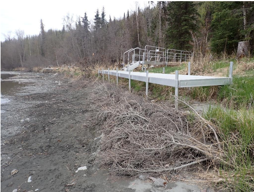
Figure 3. Post-construction looking downstream at site 202333, May 2024.
