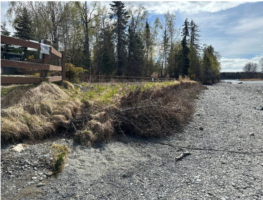
Figure 5. Post-construction looking downstream at site 202427, May 2025.
