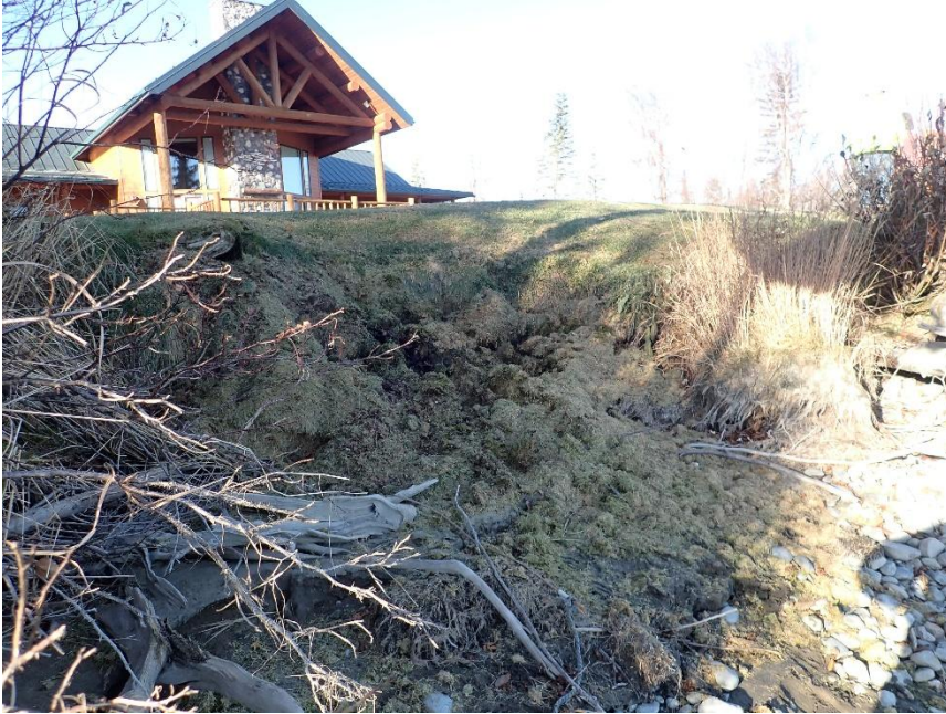
Figure 12. Pre-construction looking downstream at site 202526, October 2024.
