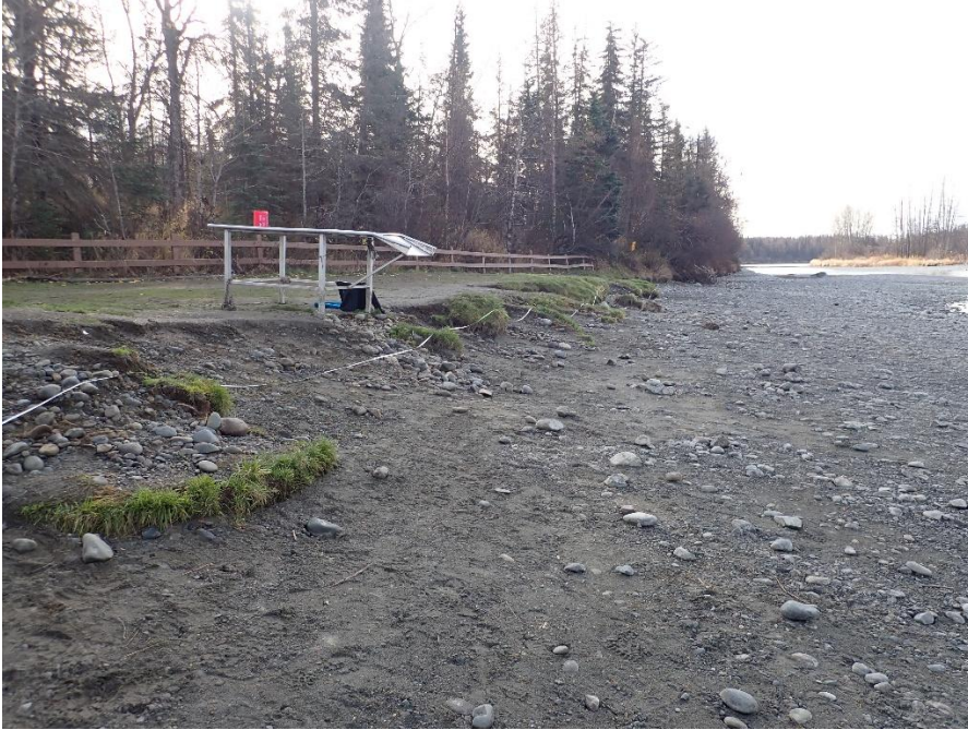
Figure 4. Pre-construction looking downstream at site 202427, October 2023.
