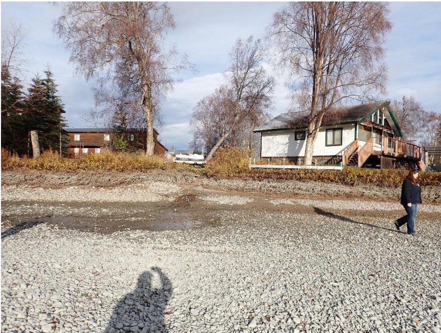
Figure 17. Post-construction looking at the bank at site 202341, May 2023.
