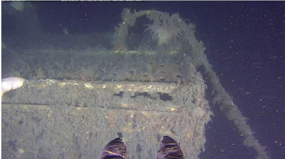
Image 2. ASLC A Line “Pig Trap” on intake, courtesy Global Diving & Salvage, Inc. 5/7/2026
