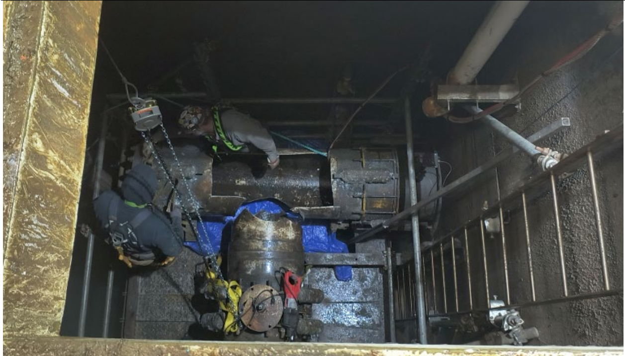
Image. AMI crew in process of removing damaged pipe to be replaced.
