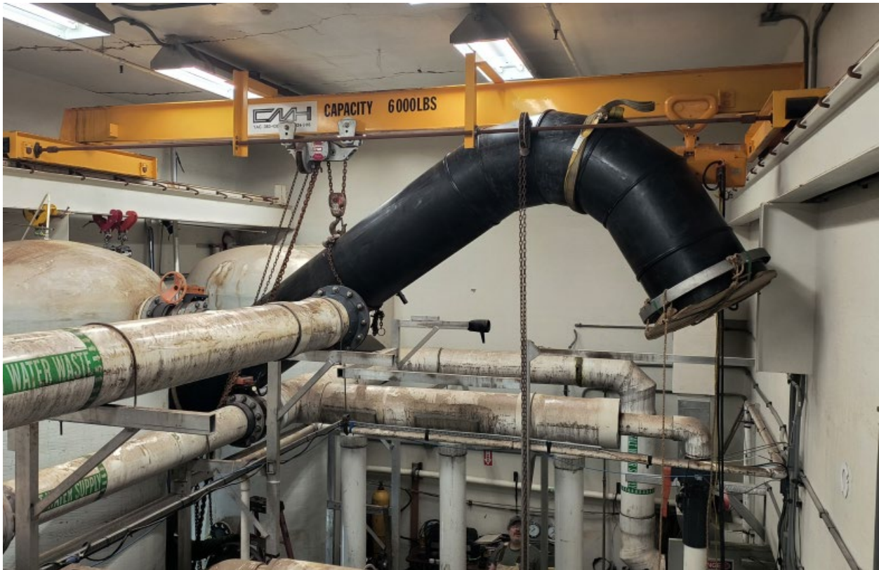
Image. Siphon downcomer section proved to be slightly too large to install into well, requiring an additional couple be used to complete installation.
