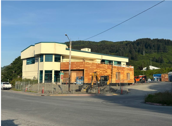
Mid construction photo with first floor addition framed and dried in.
