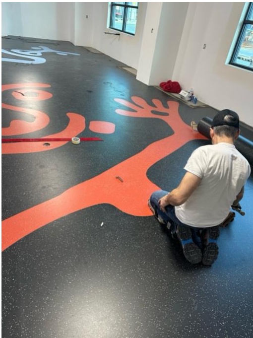
Installation of resilient flooring for the Canawik workshop space, featuring artwork designs.
