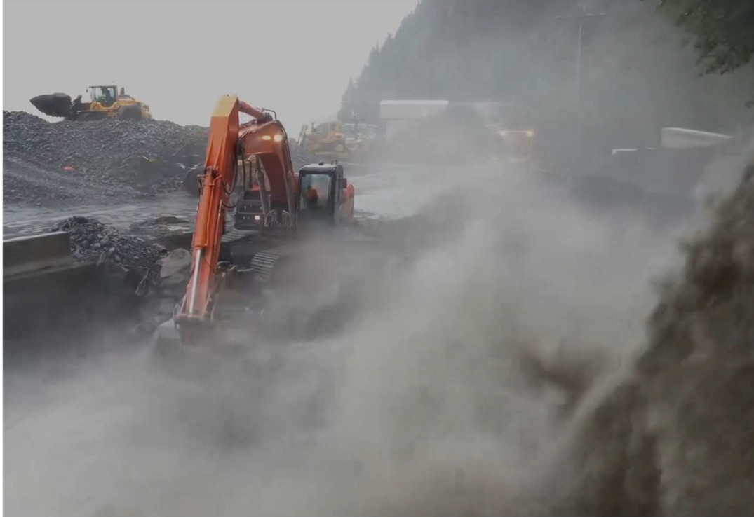
Image 2. An excavator removes sediment from the Lowell tunnel outfall directly adjacent to the ASLC fresh water pumphouse August 8, 2024. Photo credit James Unrein.
