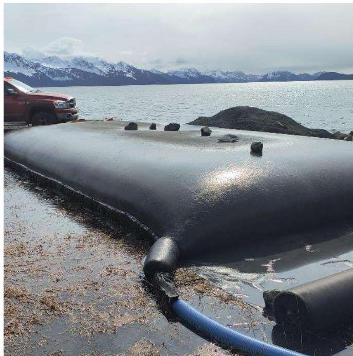
Image 4. One of four sediment collection bags that were used to contain dredge materials and filter process water.
