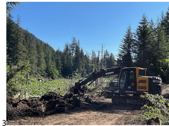
Figure 4. USFWS equipment operator at the Windy Bay Culvert construction site. July 2024.
