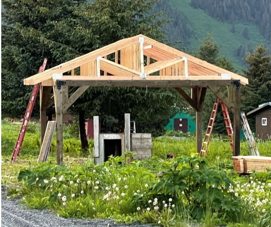
6.1 NSC Smokehouse Construction
