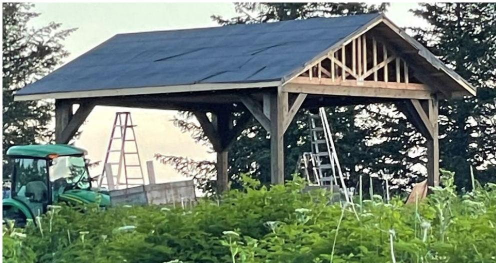
6.2 NSC Smokehouse Construction 2
