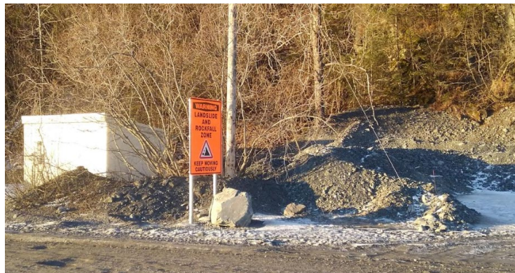
Figure 8. Freshwater Pumphouse and adjacent gravel berm on city property.
