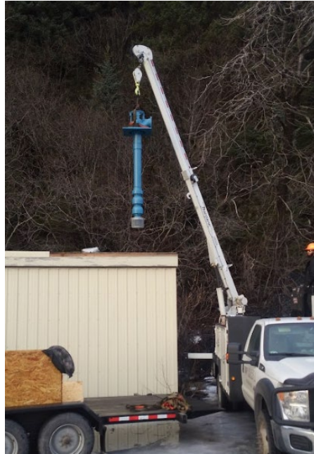
Figure 7. DXP Installing new Goulds vertical turbine pump.
