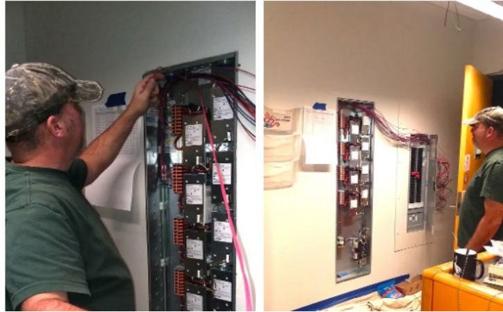
Figure 1. Trane subcontractor wiring new lighting control relay panel.
