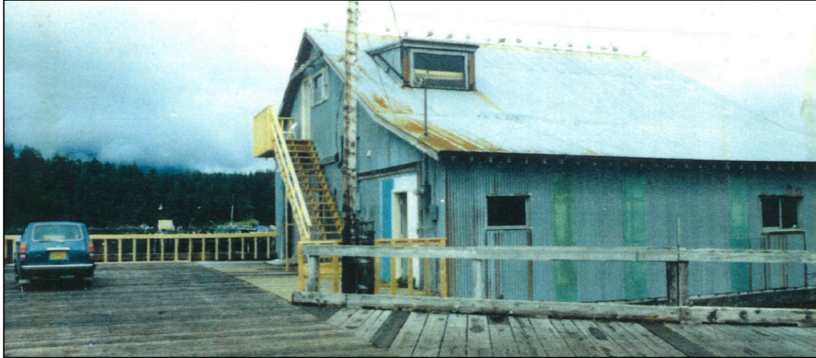
Figure 1. PWSSC (circa 1989): converted fish processing building.
