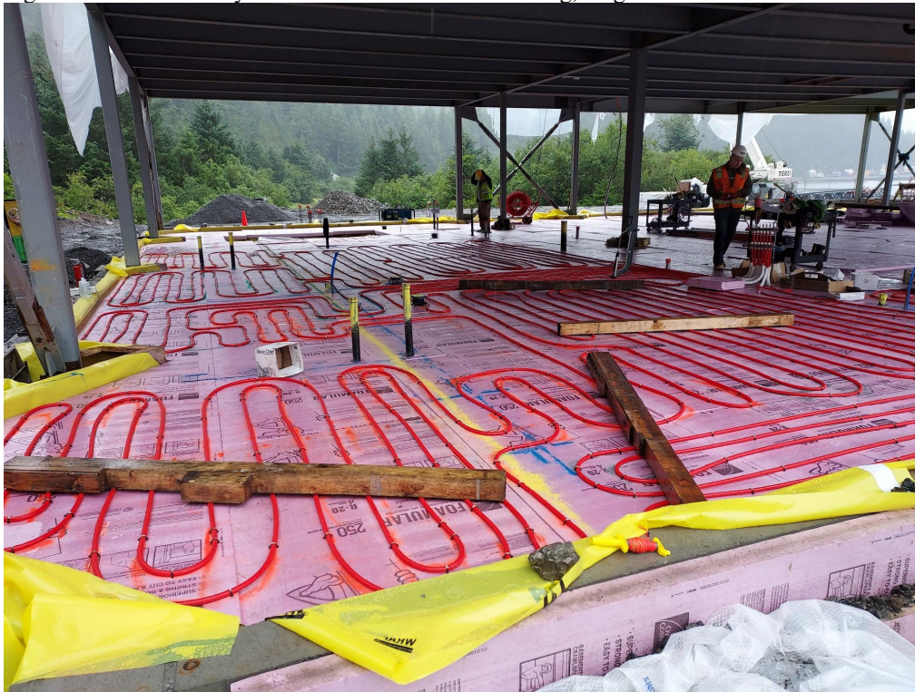
Figure 5. Radiant heat system installation in main building, August 2021.
