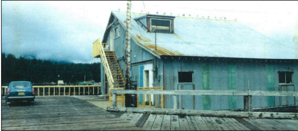
Figure 1. PWSSC (circa 1989): converted former processor & mechanic shop building.
