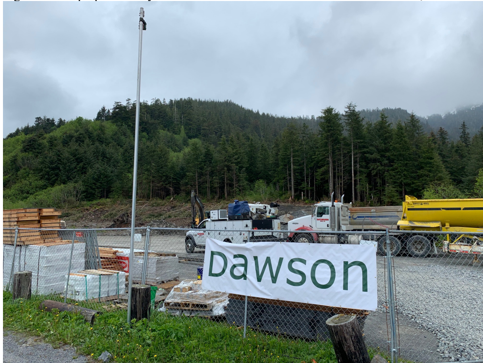
Figure 4. Site preparation by Dawson Construction and Southeast Earthmovers, June 2021.
