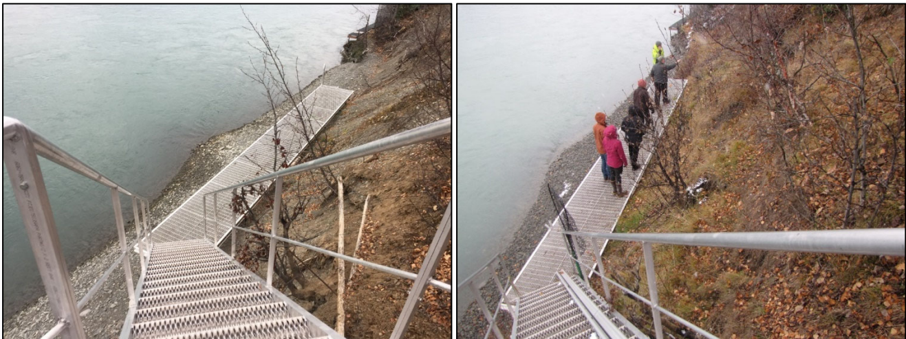
Figure 4. Photo on left is a pre-construction photo, 2017, notice bare gravel on the slope. Right photo was taken in 2019, notice complete vegetative cover of grass and planted trees on the slope after three growing seasons.
