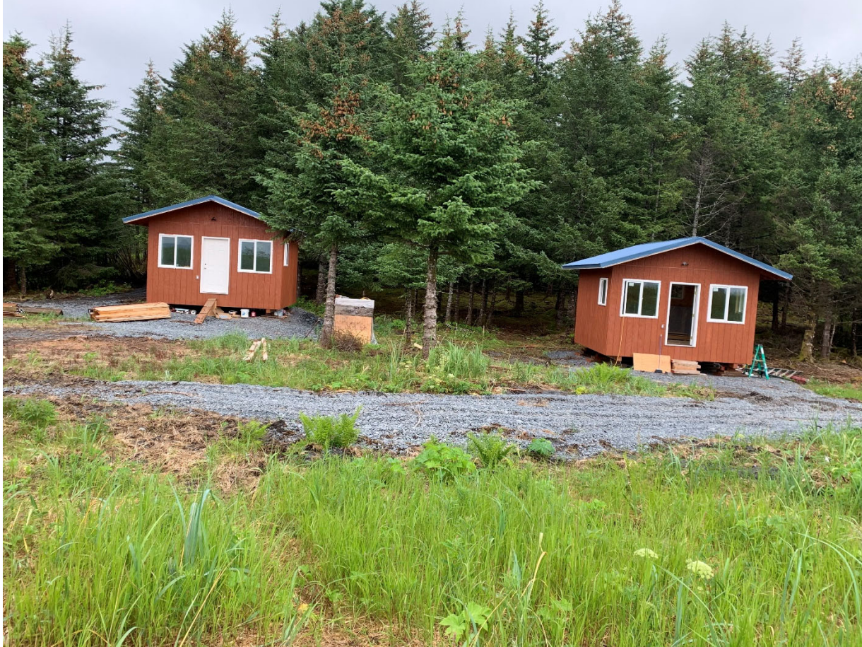
Nuchek Facilities - Beach View Cabins 1 & 2
