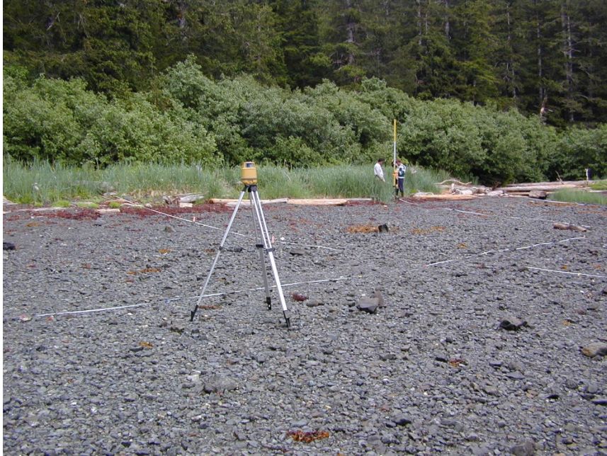
Laser level in foreground set at MHWL. Finding top of column in background with stadia rod/receiver.
