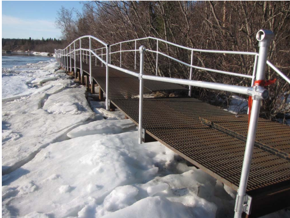
Figure 2 - Existing Walkway to be Removed (April 27, 2012)
