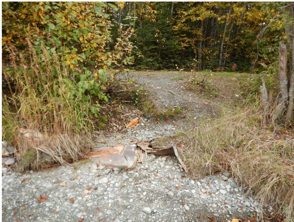
Figure 3 - Trampled Riverbank and Metal Debris at the Project Site (September 18, 2018)
