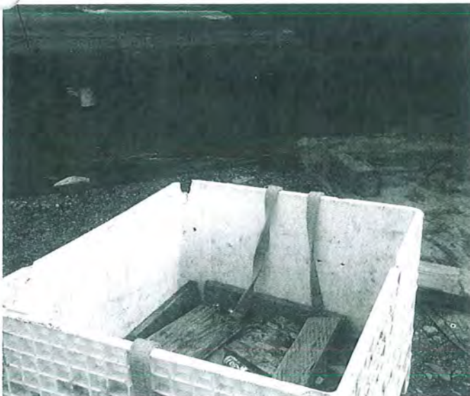
PHOTO 7: DEBRIS BIN, TARP BMPs
