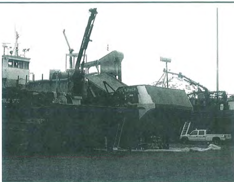
PHOTO 10: BOATS IN YARD, WORK IN PROGRESS
