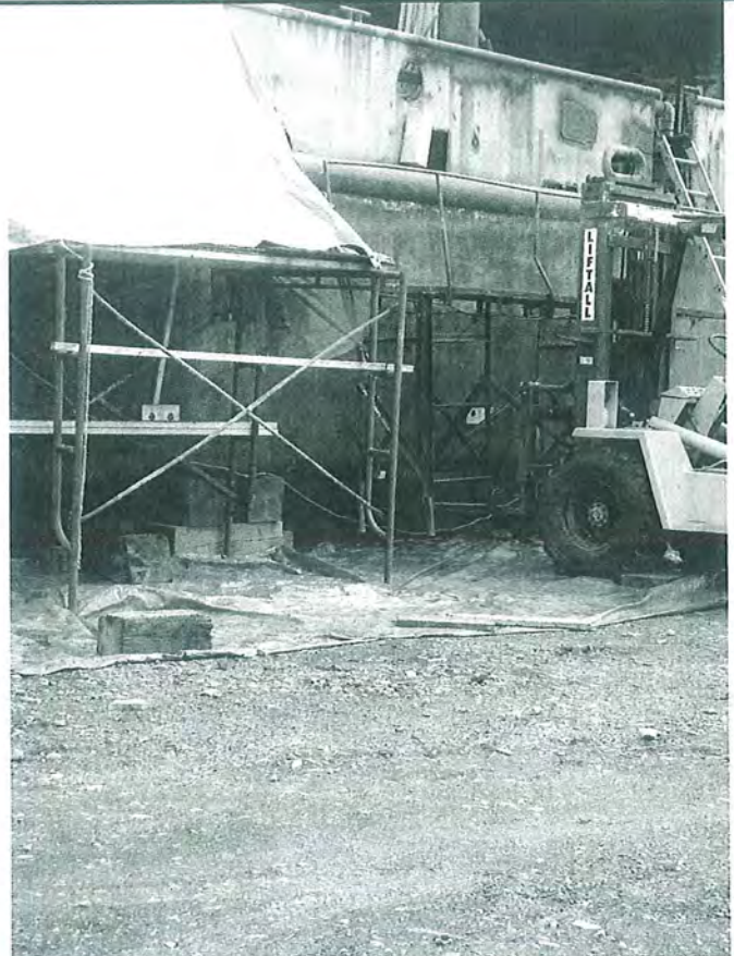
PHOTO 6: EXAMPLE OF WORK IN PROGRESS, TARP BMPs
