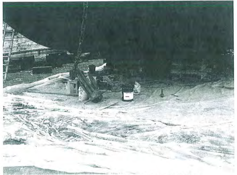
PHOTO 8: EXAMPLE OF WORK IN PROGRESS, TARP BMPs
