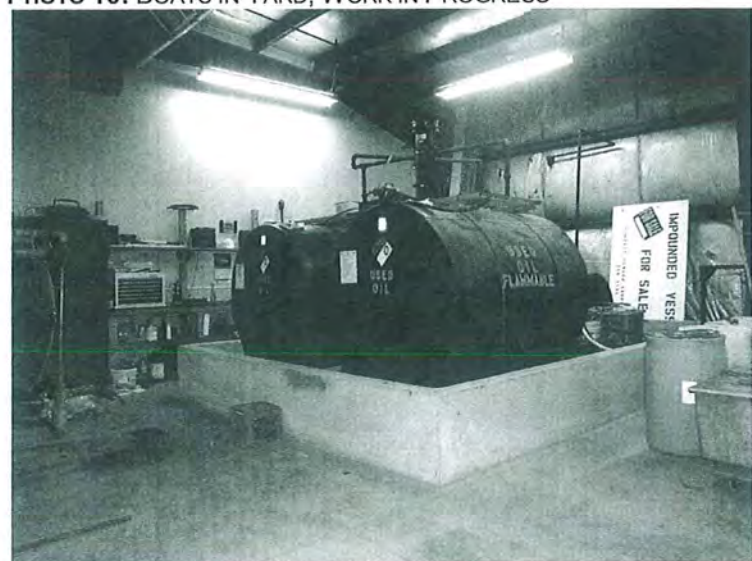
PHOTO 12: USED OIL TANKS INSIDE OF SHOP
