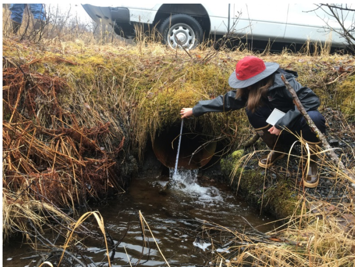
Photo 1: Perched culvert on a Battery Creek tributary
