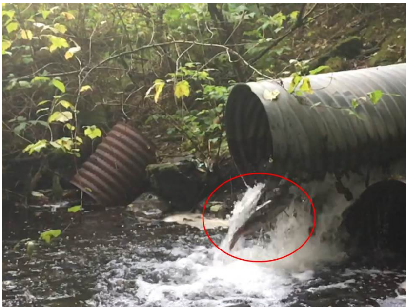
Photo 4: A coho salmon failing to pass a perched culvert at Boy Scout Lake outlet
