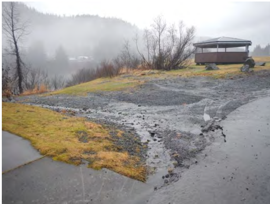
Former snow storage site upslope of Odiak Pond. January 2015
