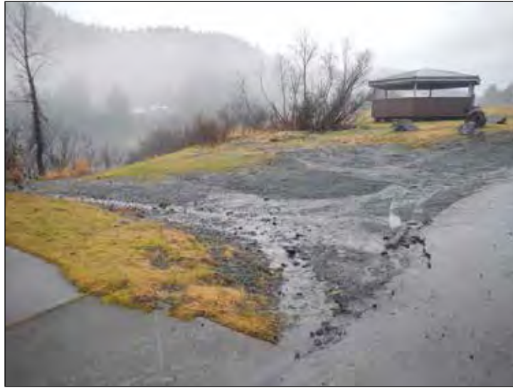
Snow storage site on the bank of Odiak Pond in January 2015. Melting snow carried sediment and adsorbed pollutants to coho salmon habitat in the pond.
