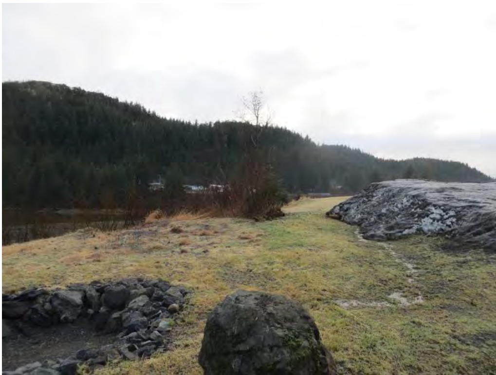
Snow storage V-swale in use. Note trickle path of snow meltwater draining to sediment trap in lower left foreground. January 2016
