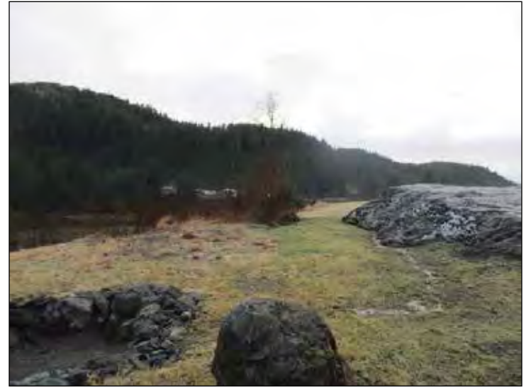
Snow stored in new V-swale, with melting snow draining to sediment trap. Sediment will be deposited in this basin before melting snow drains to Odiak Pond.
