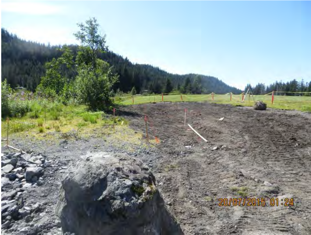
Site grading to form V-swale snow storage site. Pavilion was moved to the right. Site design originally called for wider swale, but we opted to retain vegetation on the left side for greater filtration. July 2015
