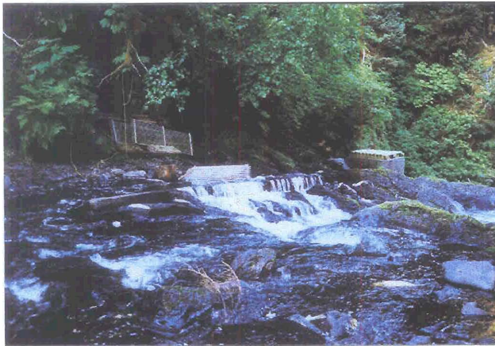
Figure 7. Photos of the third bypass at Little Waterfall Creek, with addition of aluminum resting tanks, reduced steep pass grades (a), and also showing exit channel diversion wall (b), which prevents salmon from being washed over falls.
