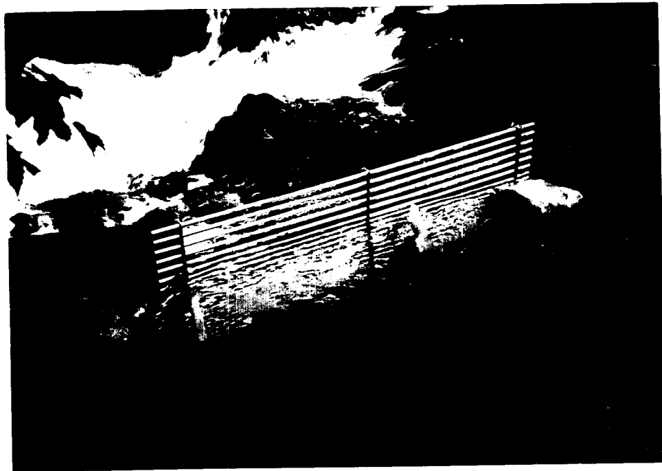
Figure 6. Photographs showing the use of aluminum picket panels to prevent “backwash” of salmon over the waterfall at Little Waterfall Creek, 1996.
