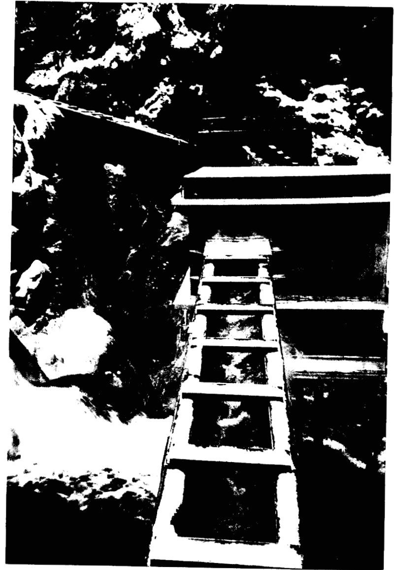
Figure 9. Modified barrier bypass at Little Waterfall Creek showing additional resting pools, and staggered steepass sections.
