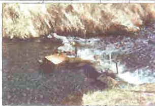
Plate M - Kametlook River water intake boxes are installed upstream approximately 50 feet from the egg boxes.
