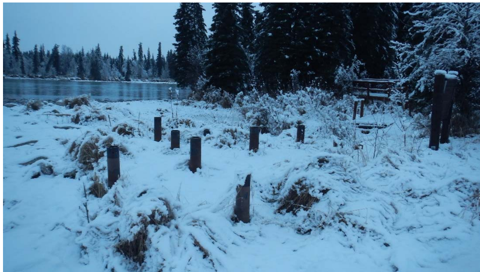
Figure 1 - Location of Previous Elevated Walkway (November 9, 2017)
