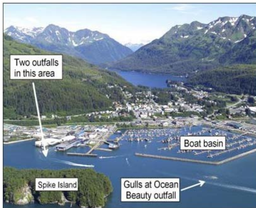
Fig. 4-3. The seafood processors in Cordova discharge ground waste via underwater pipelines into the small channel area between the Small Boat Basin and Spike Island. Thousands of gulls are attracted to the discharge plumes. When not feeding on the waste matter, the birds gather on the docks and roof tops, and in their abundance create a general nuisance with regard to public health and sanitation issues.
