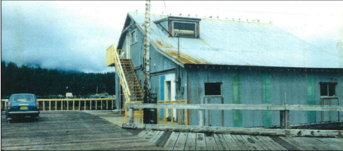
Figure 1. PWSSC (circa 1989): converted fish processing building.
