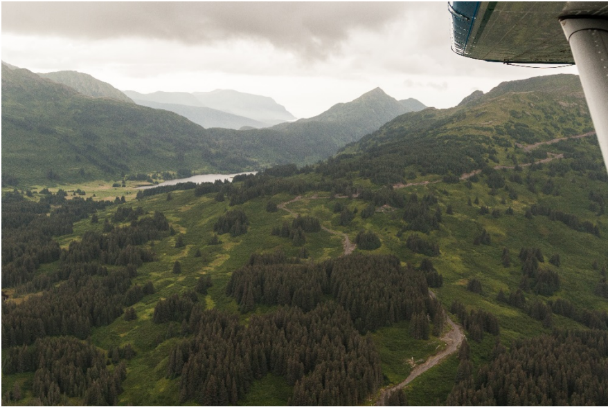
Photo: Logging road built to the edge of the subject property
