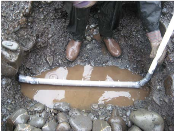
Figure 6: Photo of a 1.0 m trench with the manifold placed parallel to the shoreline before refilling the trench. A more rigid system is being proposed for the delivery of chemicals in this study.
