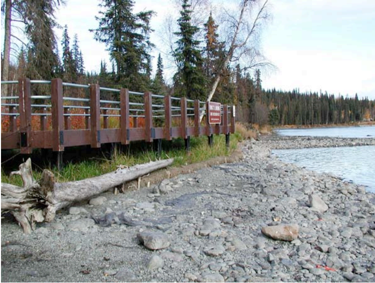
Coir Log Stabilization,
