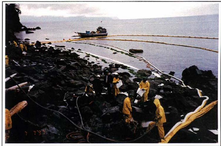
Typical boom and sorbent deployment. Shown here is LA 015C-1. Photo by J. Ginter
