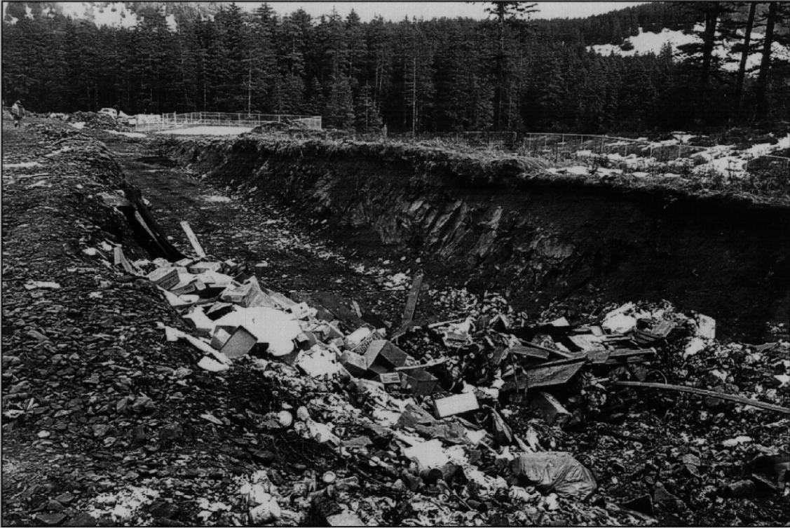
Provision for cover, controlled burning, fencing, and drainage are characteristics of a planned landfill (Ouzinkie).
