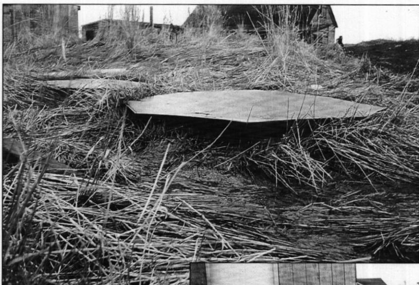
Wastewater System Failure
