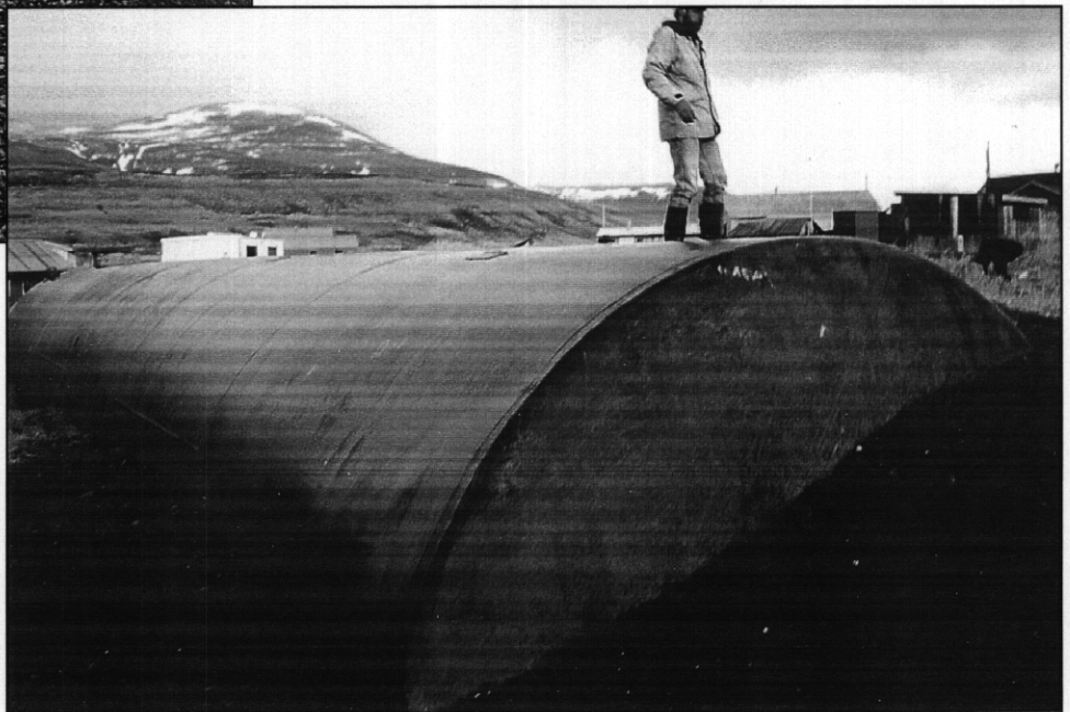
Out of service fuel tanks in Akhlok are visually unappealing and could be removed with scrap metal. Underlying soils can be checked for fuel contamination.
