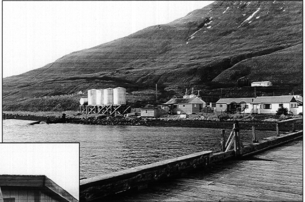
Deteriorating Old Harbor Tank Farm staged adjacent to marine resources.
