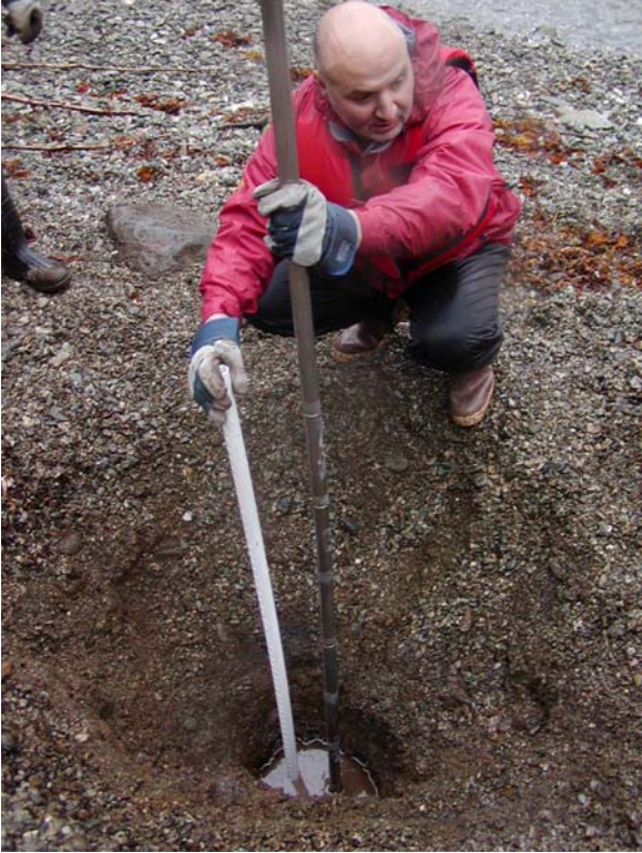
Figure 4: Placing of the water level well (the white PVC pipe) and the multiport sampling wells prior to refilling the pit.
